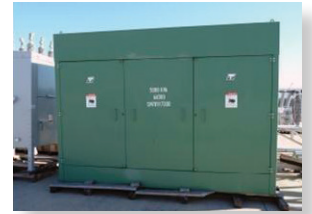
Pad-mounted transformer
