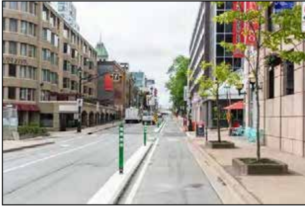
Figure 2.2.3 - Unidirectional bicycle lane on Hollis St
