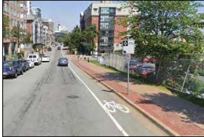
Figure 2.2.2: Painted bike lane on Lower Water Street
